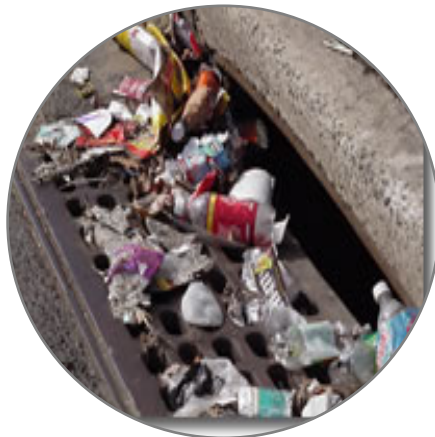
Storm Sewer System
