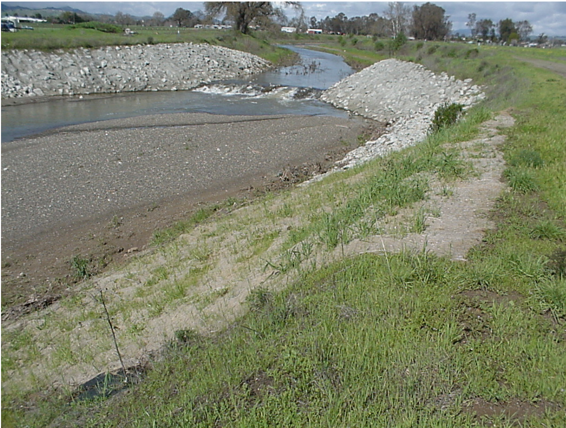
FIGURE 10:A Creek Bank Stabilization Method
