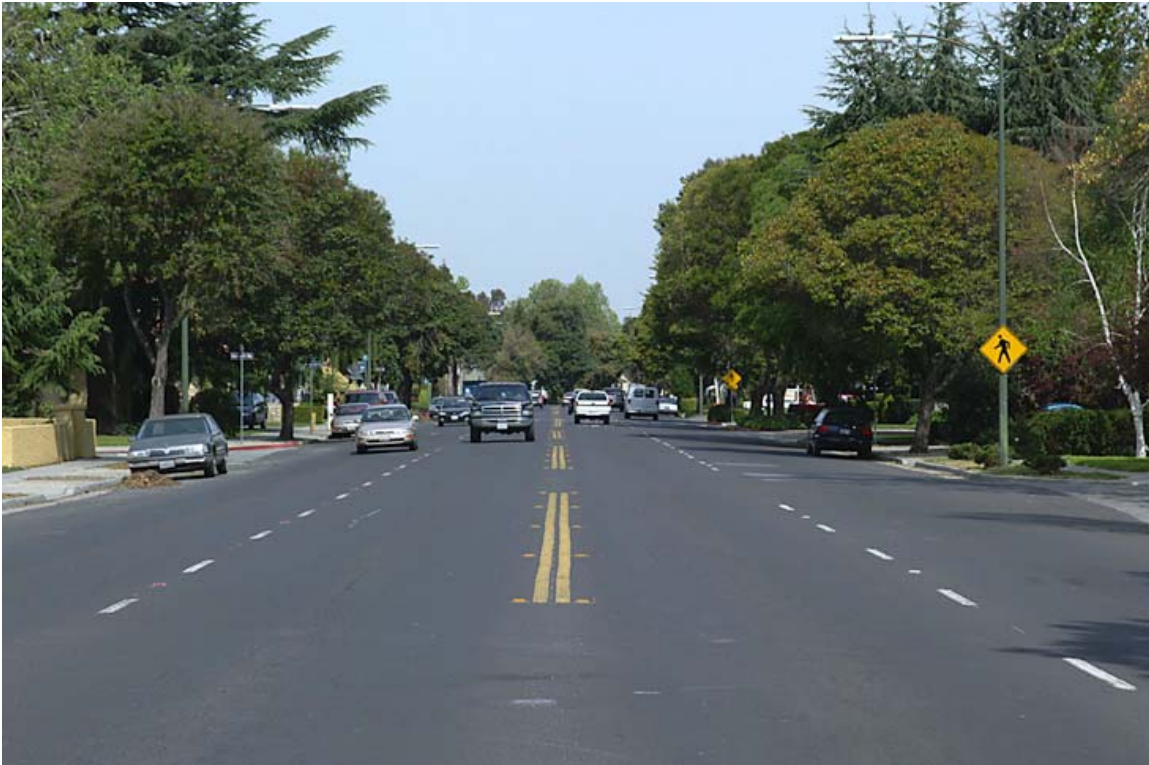
FIGURE 16:A Four-Lane Road
