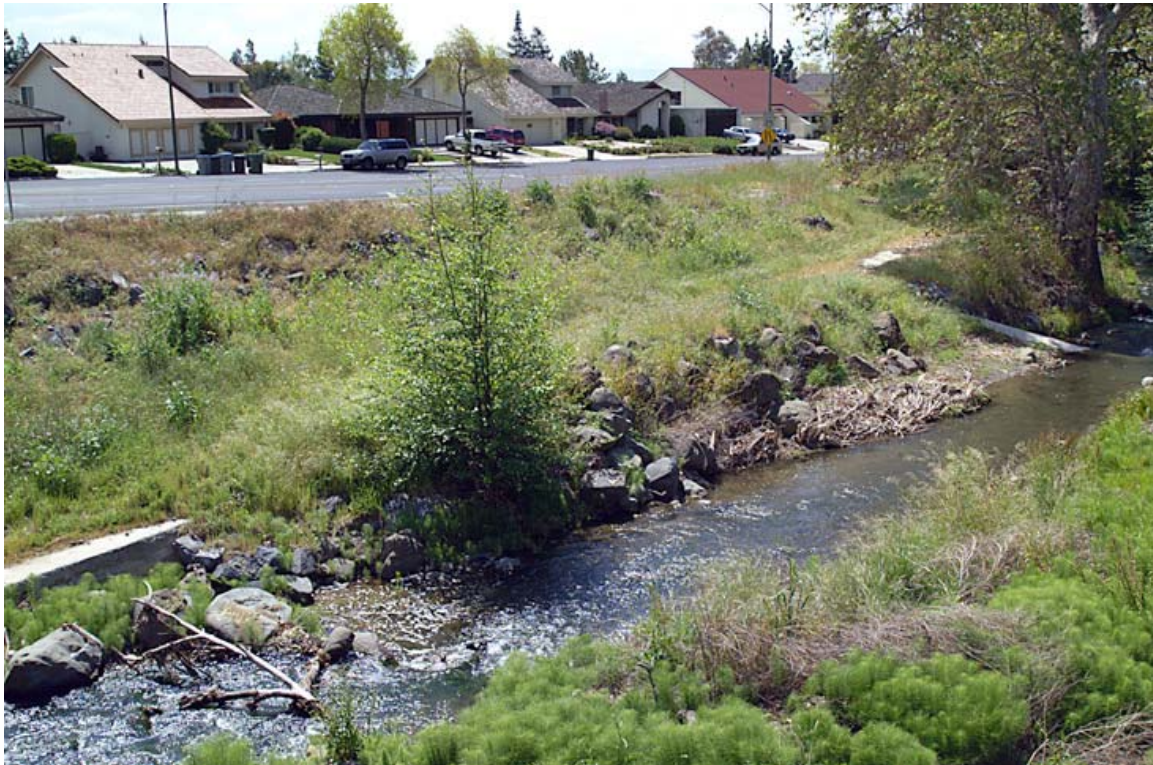
FIGURE 72: Development Along Creeks
