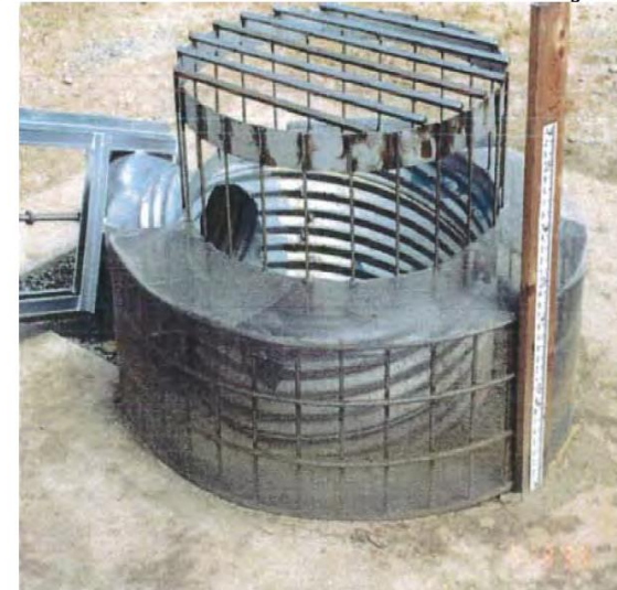
Outlet Screen - Water Quality Riser
