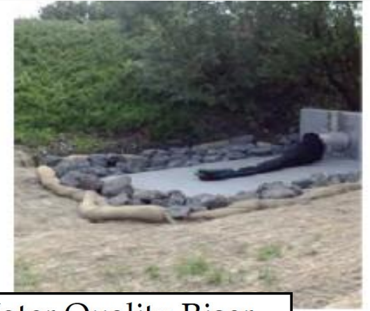
Outlet Screen - Water Quality Riser
